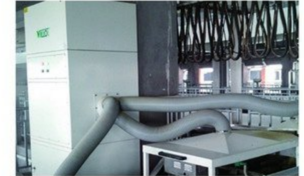
Belt transshipment point dust cleaning
