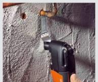
Ideal for dismantling installations that are no longer required. The E-CUT universal saw blades can be used to cut off pipes flush to the wall for subsequent filling.
